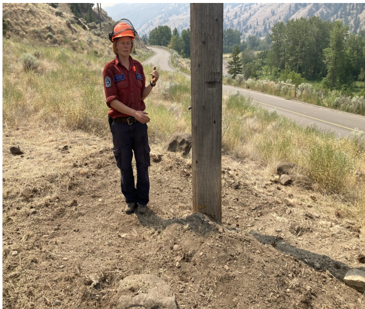
BCWS Firefighter explains how removing fuel around utility poles is a key aspect of protecting infrastructure. Brush under powerlines and laddering branches were also removed.
